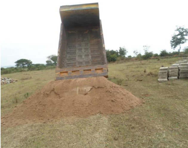
Vehicle delivering construction materials at site
