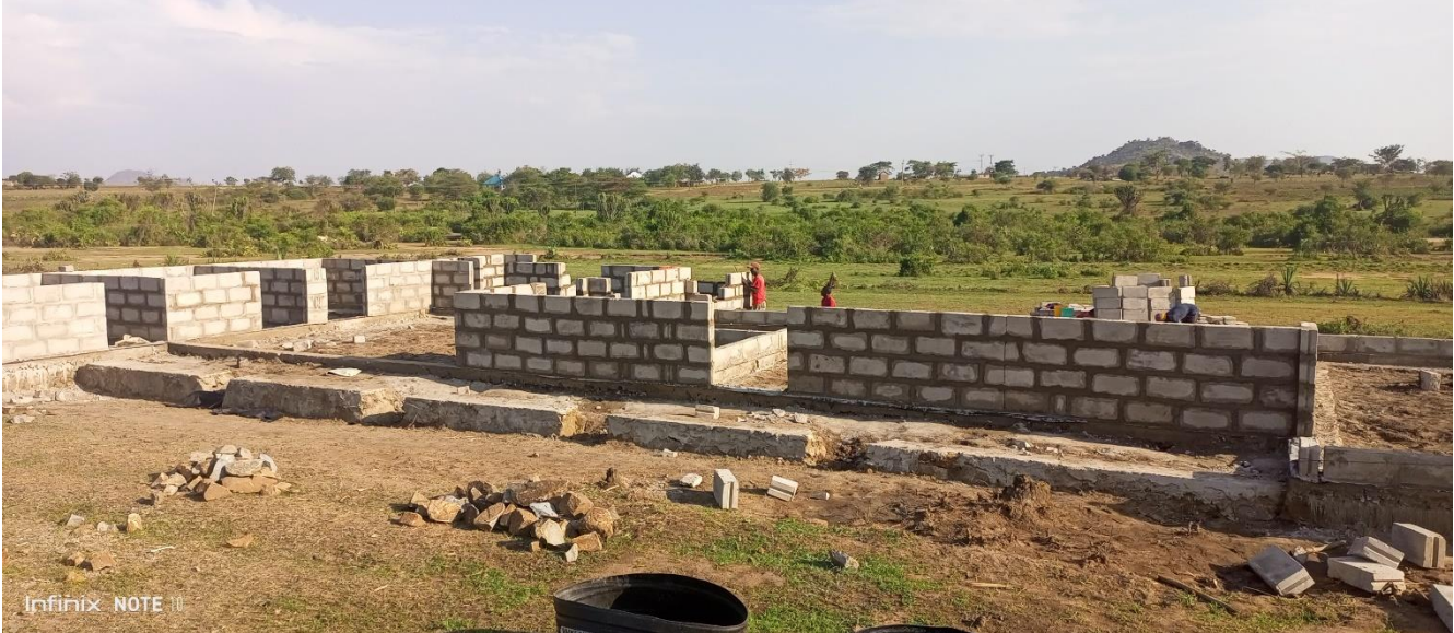
Progress of the construction of HCF at Kyamwame
