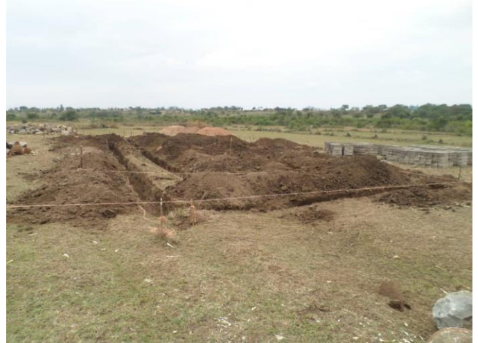
Excavated trench and material delivered at site ready to commence construction
