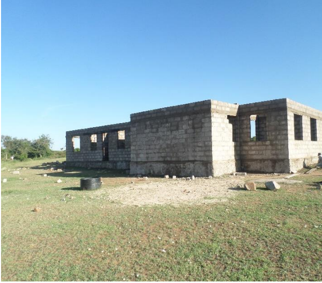
Status of the constructed HCF
