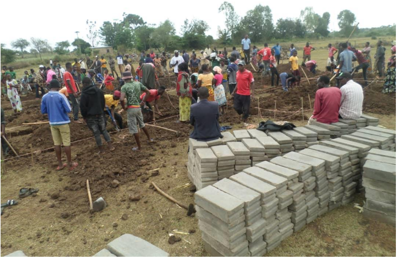
Ongoing men and women participating on construction of HCF
