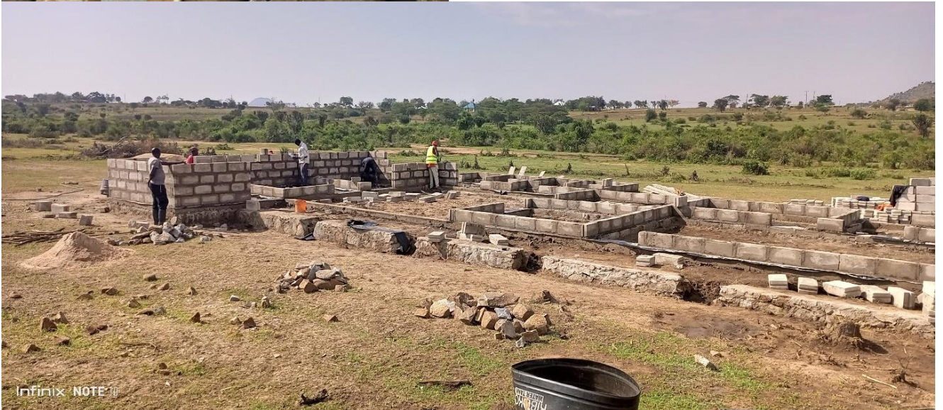
Starting of the construction of HCF at Kyamwame village, Rorya
